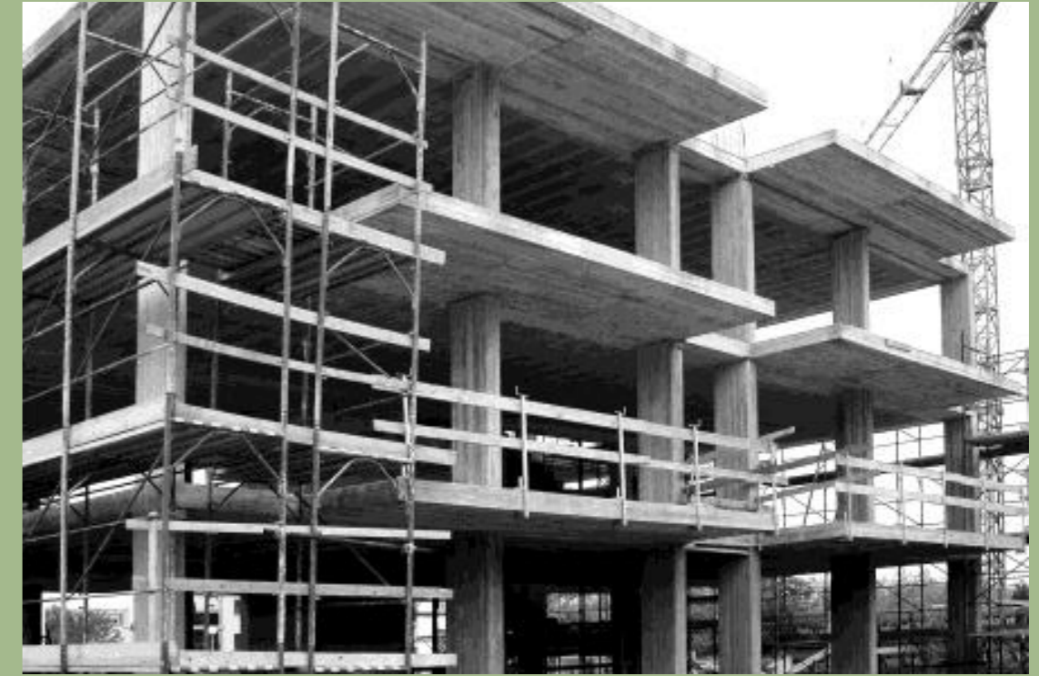
Concrete structure commonly used in housing projects [30]
