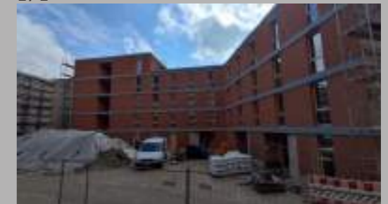
Location: Tempelhof Stage: Construction Tenancy: 200
