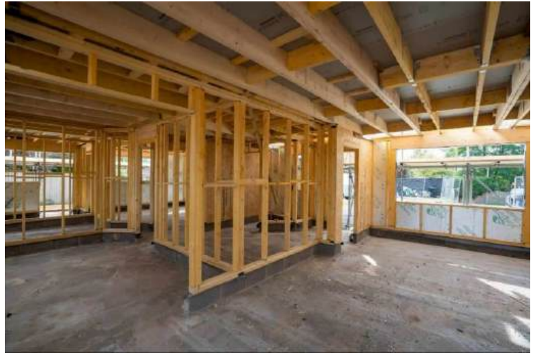
Figure 5 Timber Frame Wall Construction
