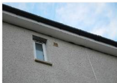
Roof Finish, mastic, cav. vent.
